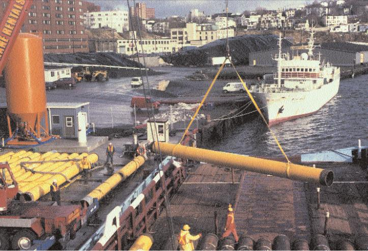
Workers load pipe onto a supply vessel in St. John's harbour. Many types of pipe, casing and riser are used in offshore exploration and production. Photo from HMDC.
